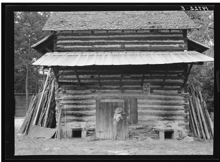
FSA caption: Tobacco barn. Person County, North Carolina. Piece of sheet iron on the left is used to cover the opening of the furnace when starting the fire (Dorothea Lange, July 1939).
